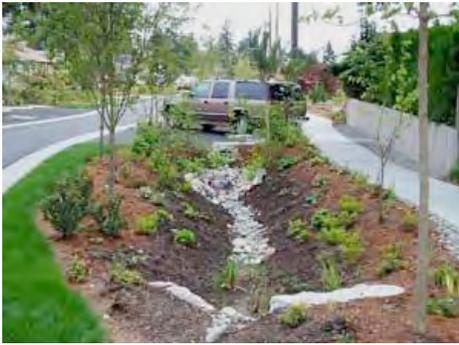
**Bioswales:** Bioswales are vegetated drainage ways that convey runoff. Typically, the subgrade of a bioswale is engineered to ensure infiltration of runoff from small rains. When big rains occur, the bioswale will infiltrate the dirty first flush of runoff and then convey excess runoff to receiving waters. Maintaining and enhancing natural drainage ways can save money by eliminating the need to install storm sewers.
