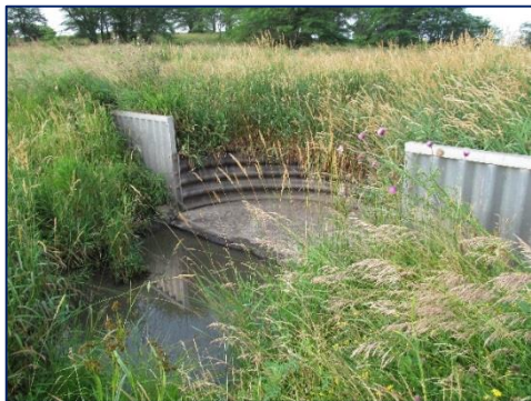
Waterway with aluminum toewall
