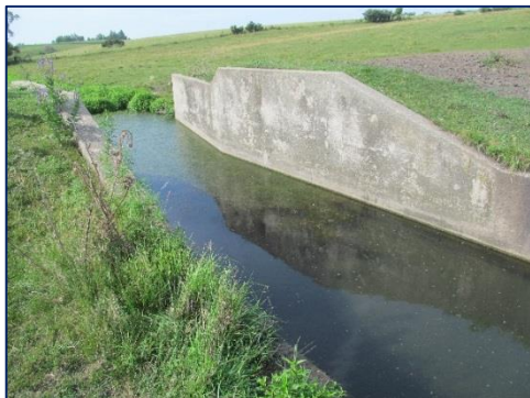
Waterway with drop box structure
